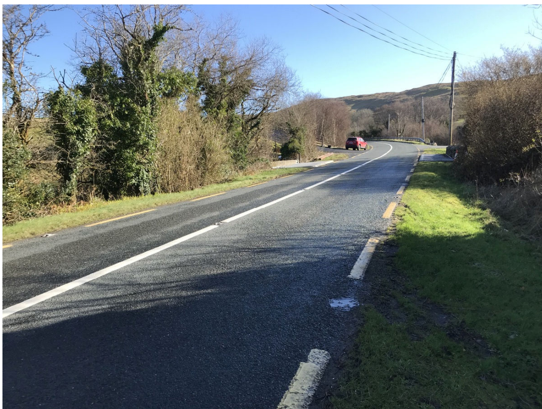
Figure 3 : View looking East
